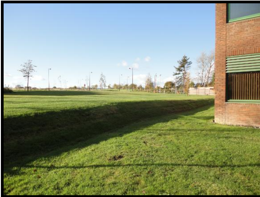
Image 4.3.1; Ground level slopes down as it nears building.
